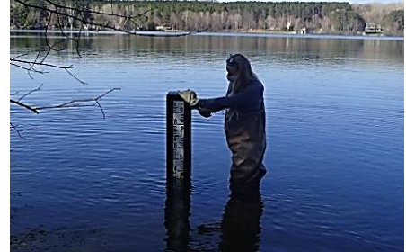
Water level gauge install at the Farlain Lake, boat launch
