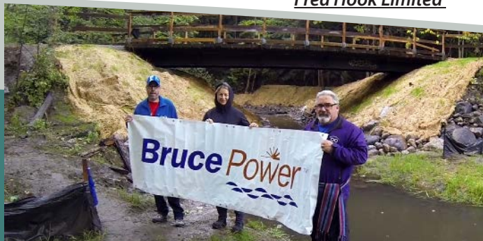
Georgian Bay Metis Council Copeland Creek Rehabilitation Project at Bridge P5
