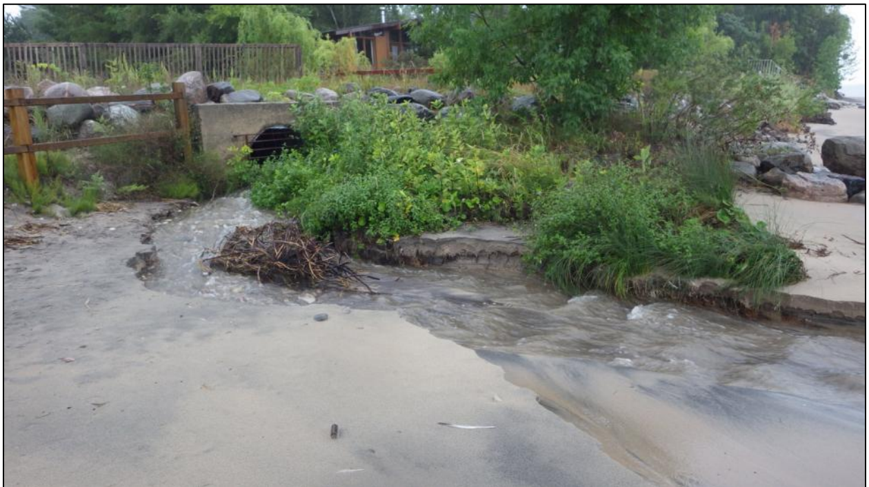
Aug 16 DB1 – Heavy rains caused large stormwater flows to discharge at the outlet, creating significant channelling; very dynamic channel.
