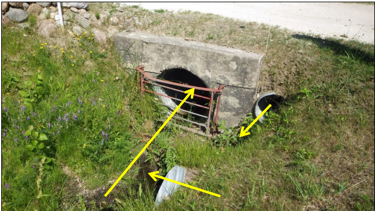
Jul 6 DB5 – Confluence showing overflow ditch culvert which flows in at this location (upper right culvert, dry), road crossing culvert (bottom, water seen flowing in during this dry period) and main culvert that goes to the manhole downstream of DB6a (upper left culvert, small amount of flow).
