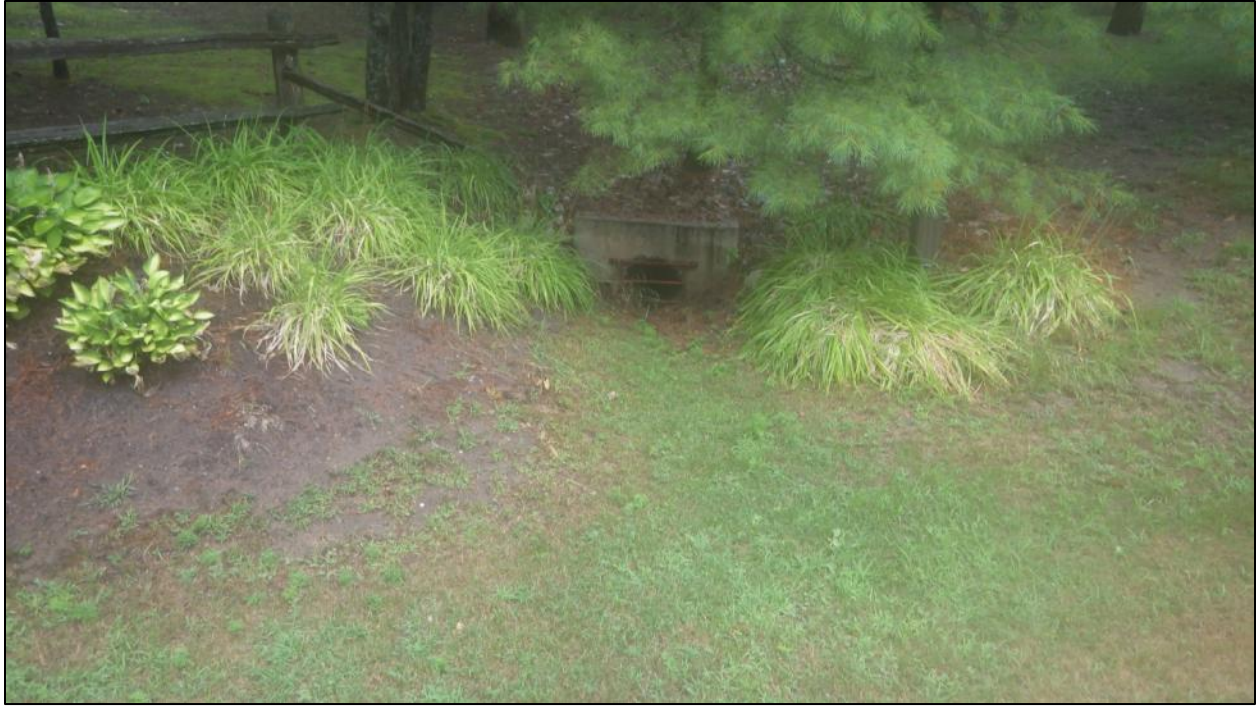
Aug 16 DB6b - No flow entering culvert despite very heavy rainfall.
