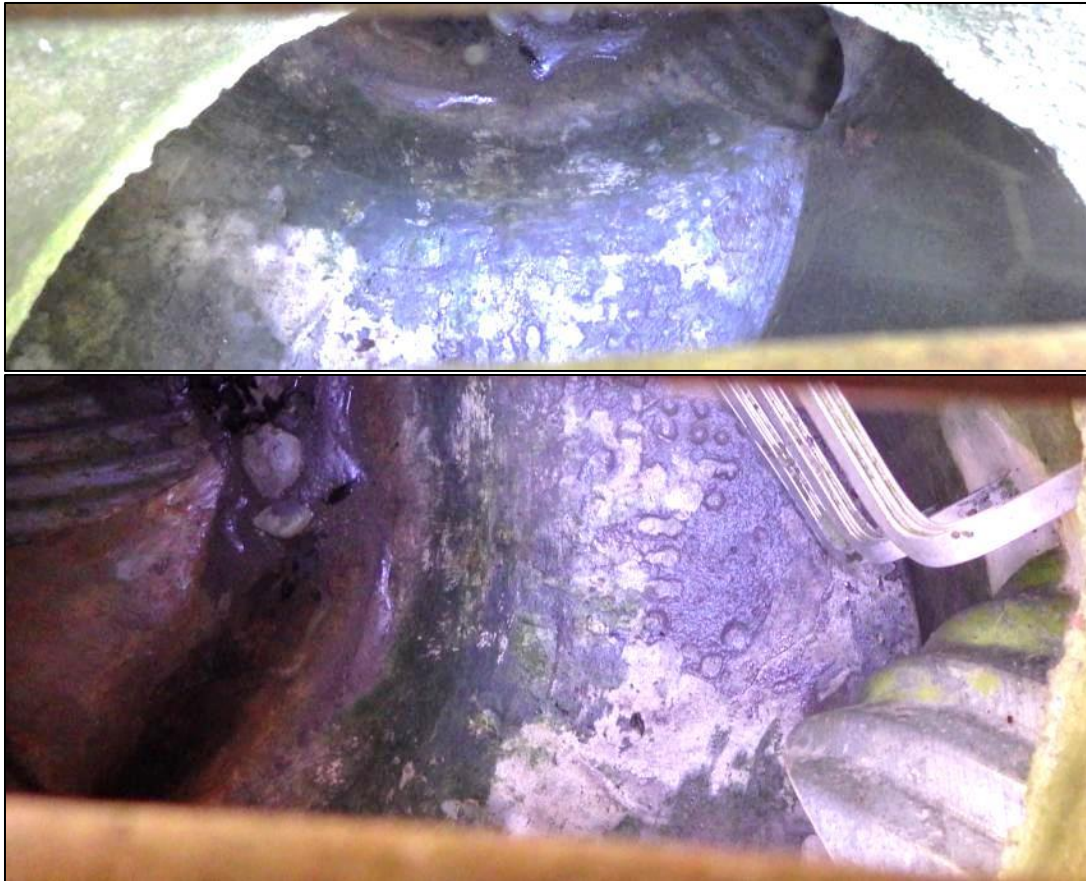
Jul 6 manhole downstream of DB6a - Water could be seen through manhole cover on both dry days (Jul 6 and Aug 3). Flow observed in culvert coming from DB5 direction (culvert in bottom photo). No flow observed in culvert coming from across the road, opposite DB6a (culvert in top photo).
