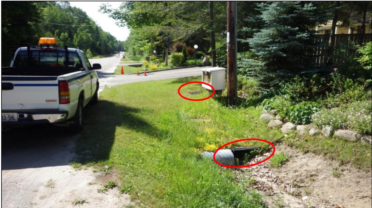
Jul 6 DB6a - Confluence of road ditch from both sides of road. After entering the rectangular culvert (foreground), the drainage disappears to manhole (circled) and onward to DB7.
