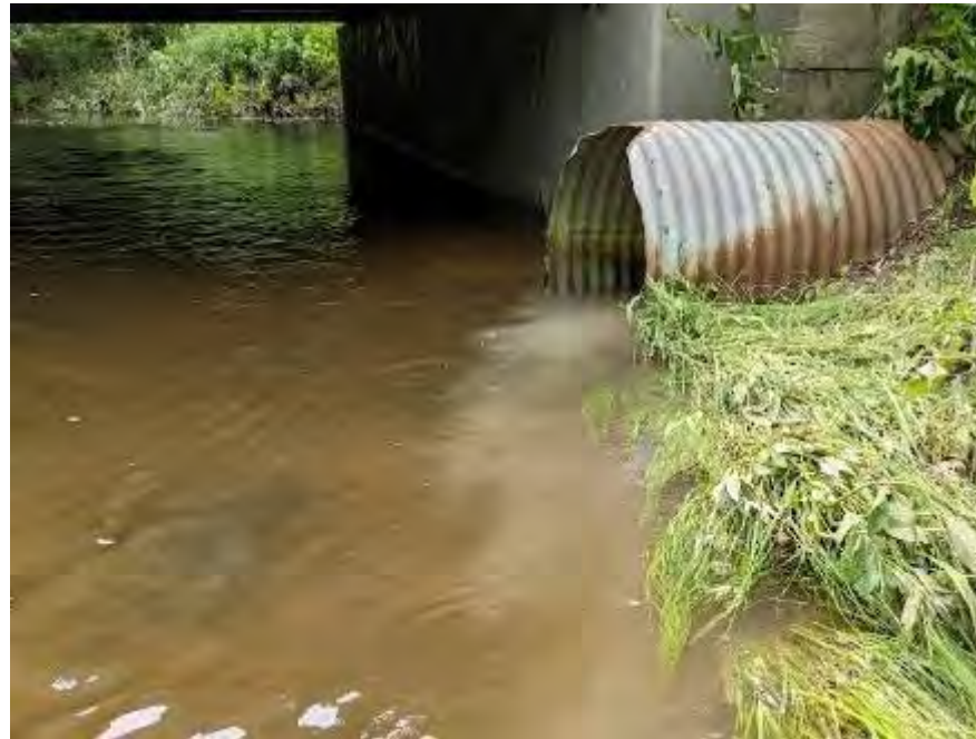
Top drain (left) and end of pipe (right) showing sediment filled stormwater entering the Wye River during a wet weather event
