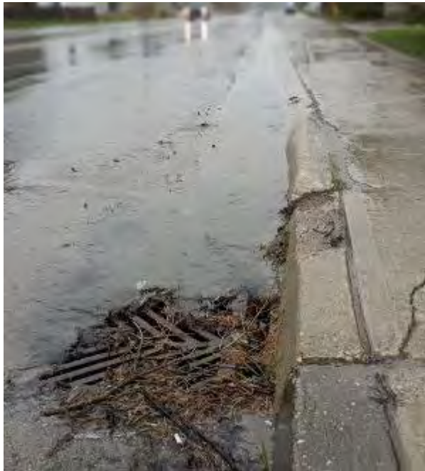
Top drain (left) and end of pipe (right) showing sediment filled stormwater entering the Wye River during a wet weather event
